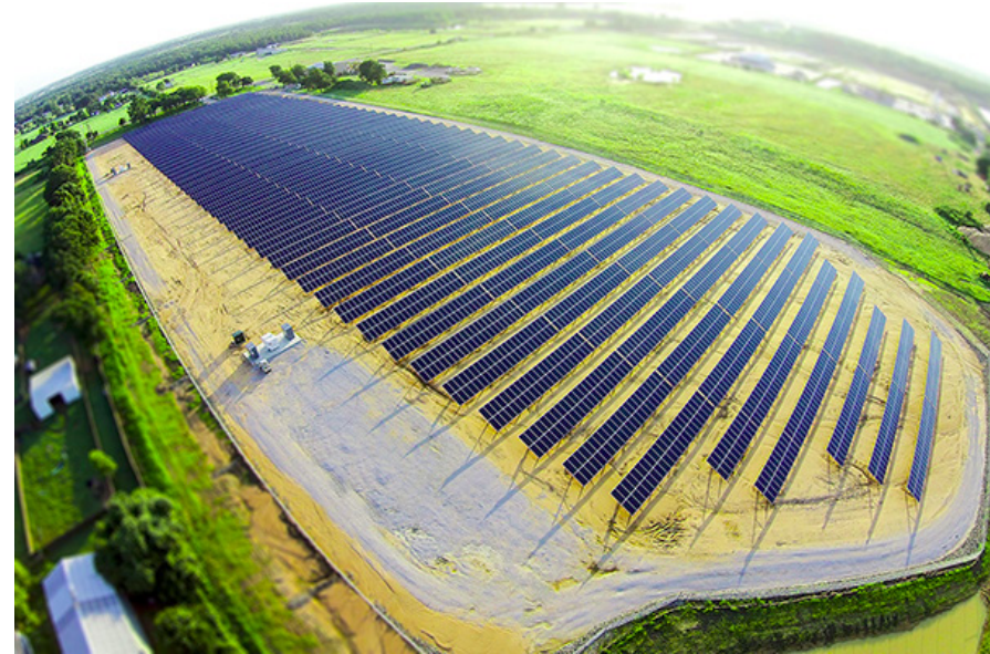
CoServ Community Solar, Krugerville, Texas (NE of Denton)
