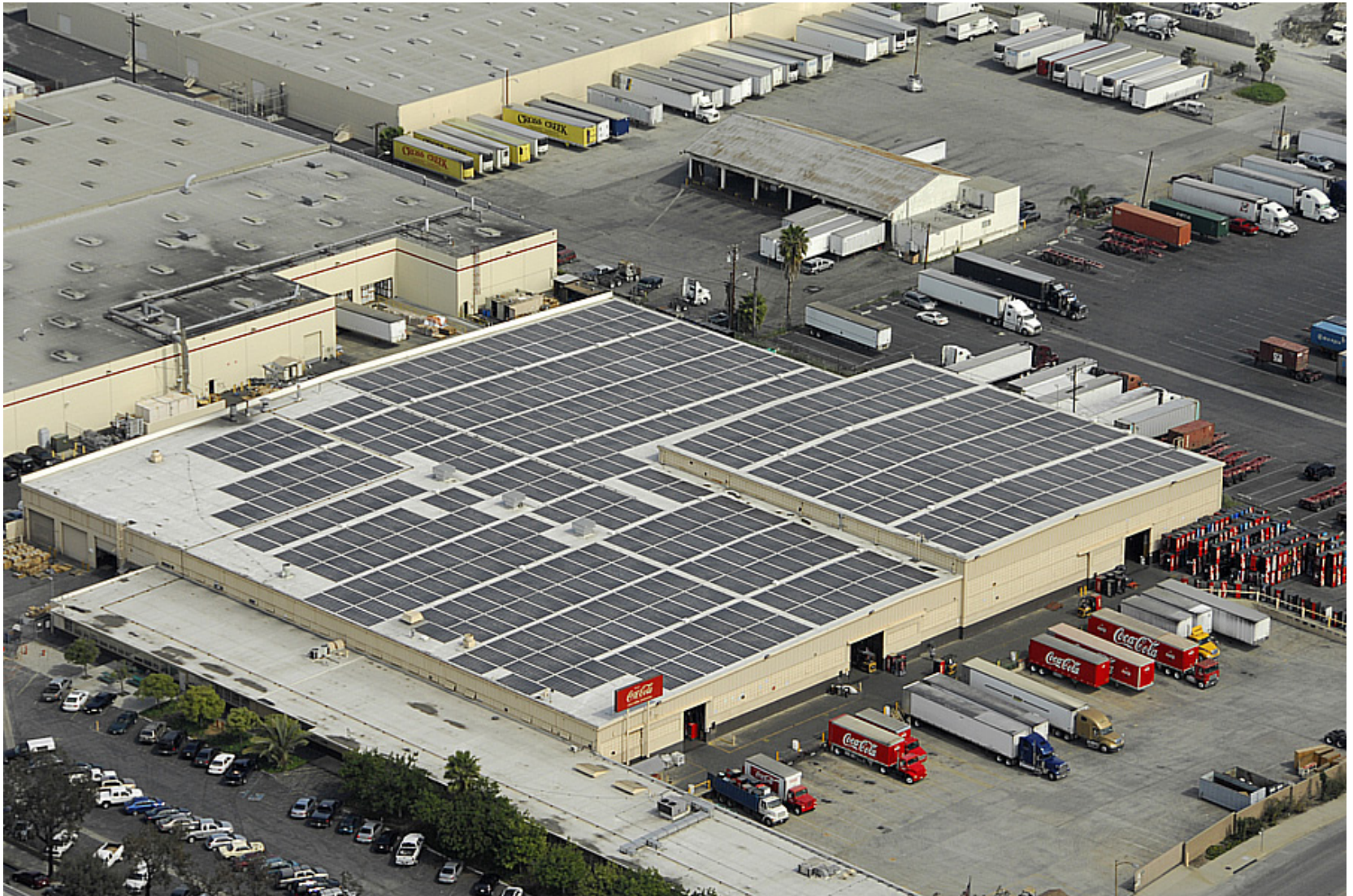
Coca Cola Distribution Center in Montebello, California (375 kW)
